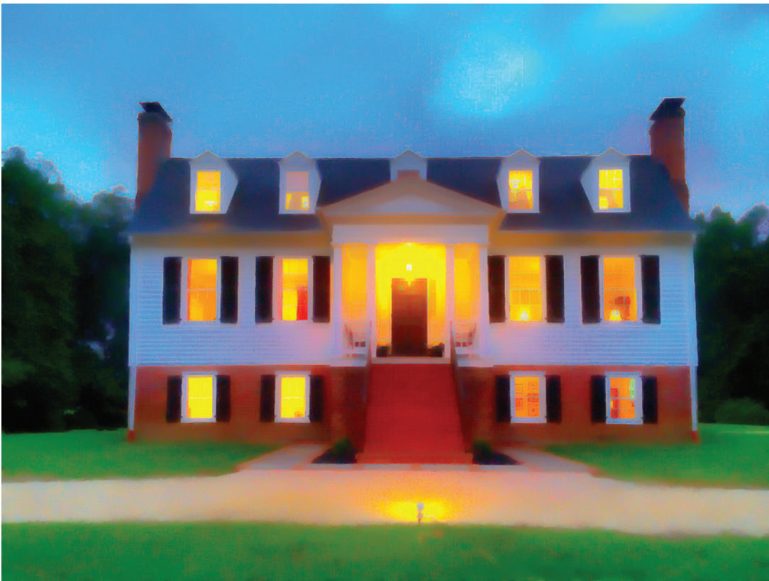
White Plains—Hanover County. Original structure dates back to 1791
